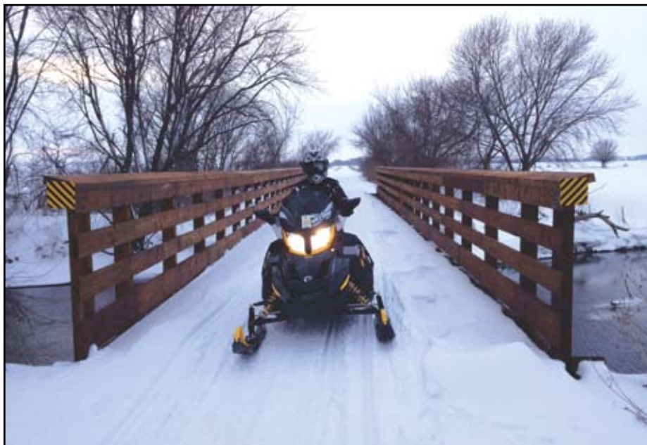
Members of the Iowa River Riders of Region 3 test out the new bridge crossing on the Rolling Prairie Trail.
