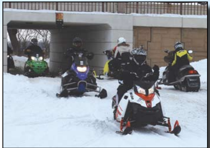
Groups of snowmobilers take turns crossing between East and West Lake Okoboji through the tunnel under Highway 71.
