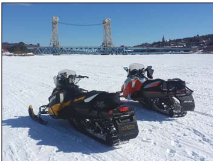
Houghton-Hancock Lift Bridge
